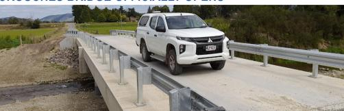
After several months of construction, Crouches Bridge is complete and has reopened to traffic. With the old timber bridge coming to the end of its serviceable life, plans were in place to replace the structure with a new bridge – comprising two 16 metre spans. The new bridge, which officially opened last month, has an increased flood capacity.
