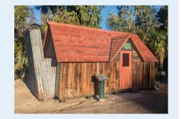
sawn totara slabs, the roof structure and roof panels have been rotting and past repair works have been done with pine.
