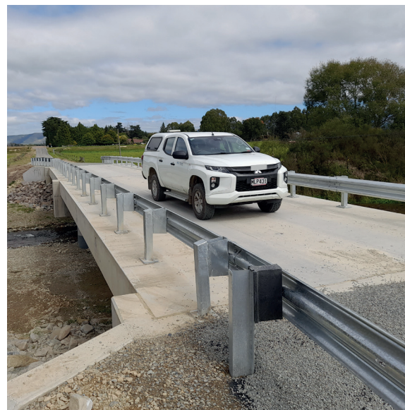
Crouches Bridge on Youngs Road was replaced with a two span concrete single lane bridge, marking the district's most substantial roading renewal project for three decades.
