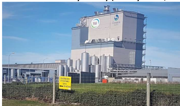
Figure 6.13 - Oceania Dairy Factory (Cooneys Road, Glenavy)
