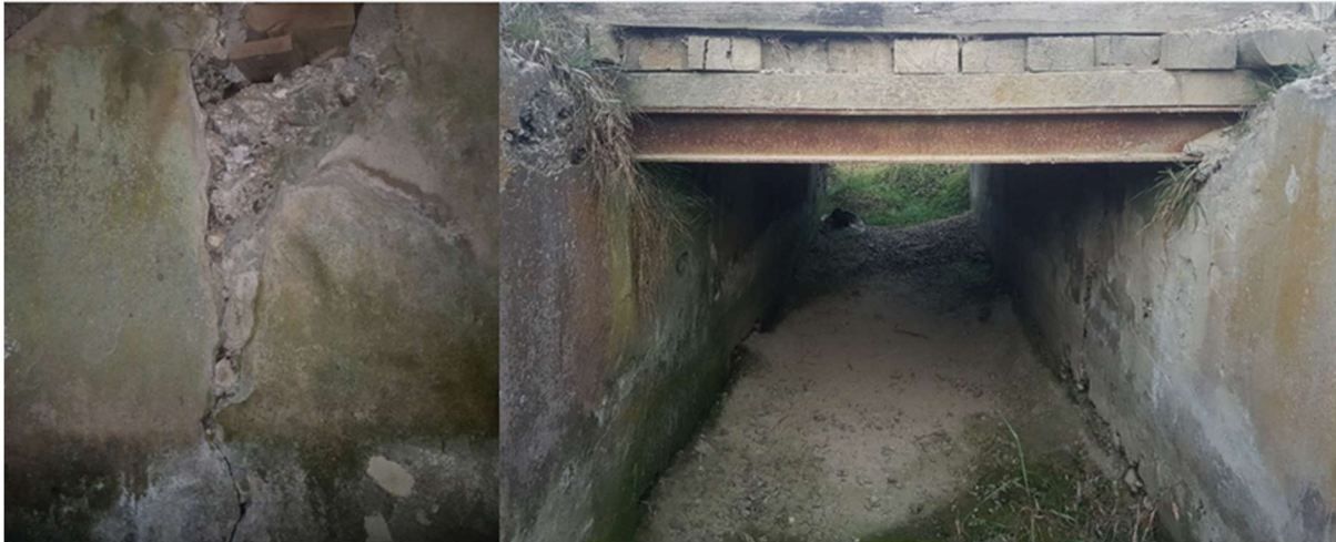
Figure 9.44 - Large Culvert Replacement - Hillboro Culvert
