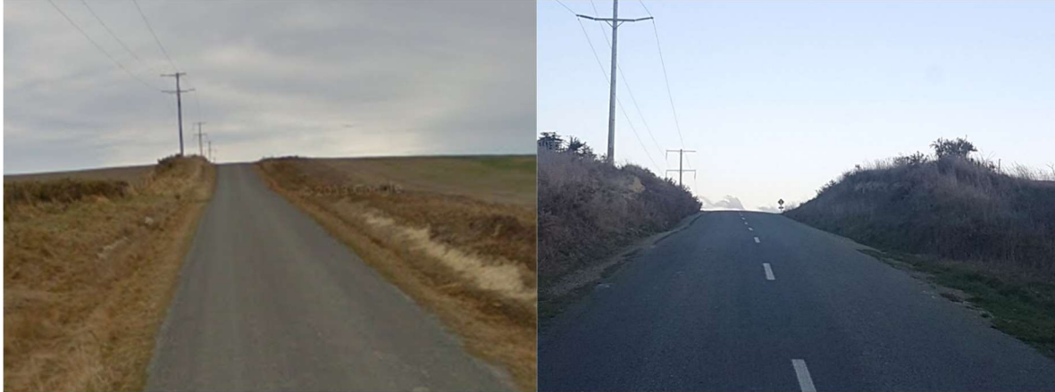
Figure 9.66 - Seal Widening Completed on Talbots Road, Blind Brow
