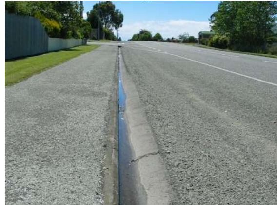
Figure 9.43 - Shallow Type Kerb and Channel
