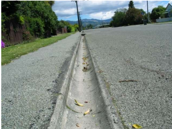
Figure 9.42 - Deep Type Kerb and Channel
