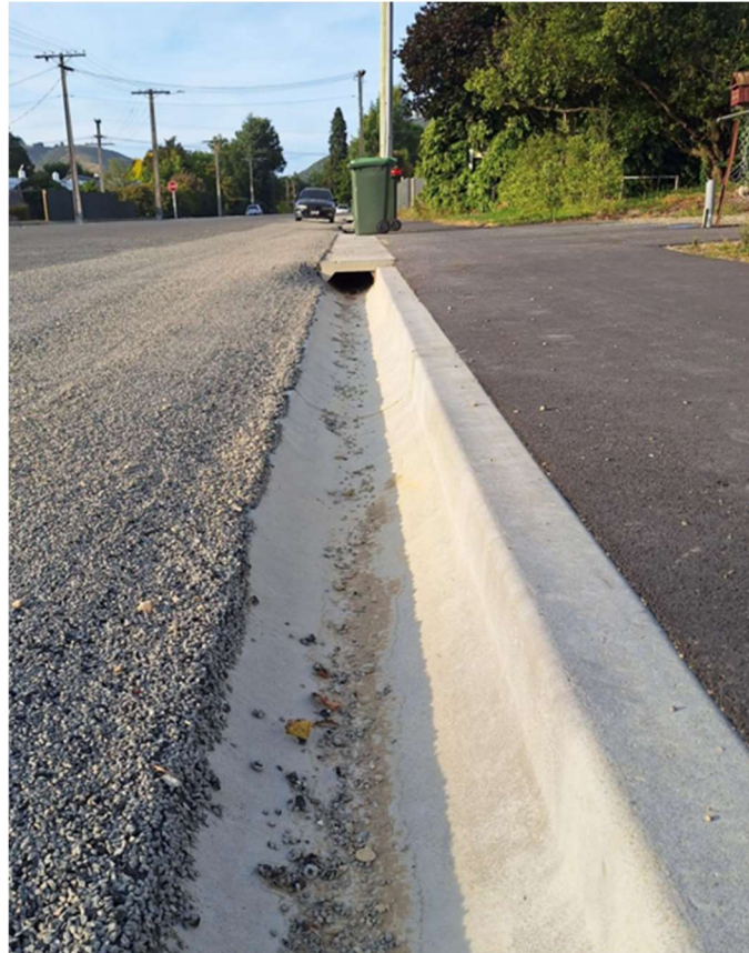
Figure 9.38 - New Dish Kerb and Channel
